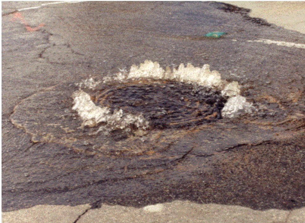
Figure 12: Sanitary sewer overflow (SSO)
