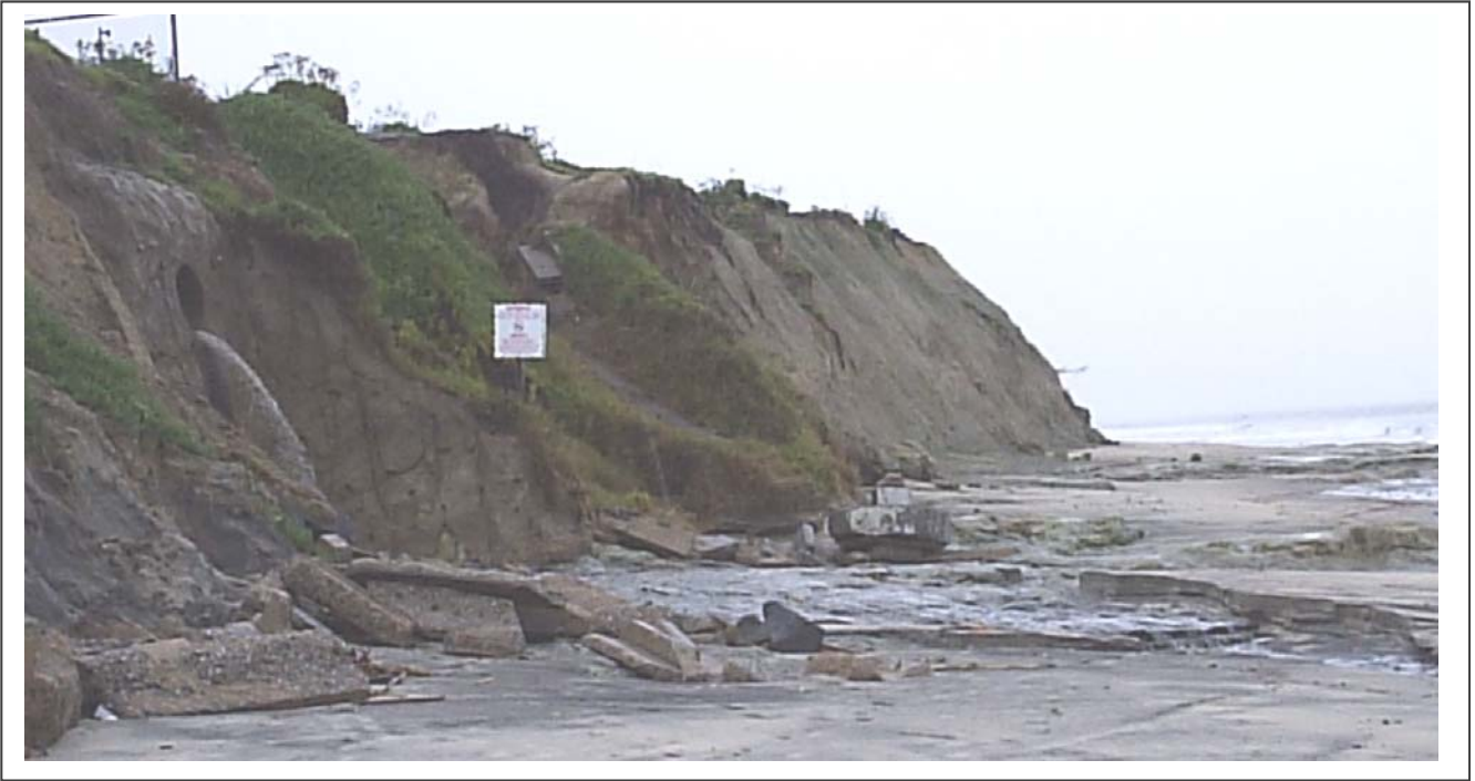
Figure 17: Wet weather flow at 15 th St. storm drain outlet in Del Mar
